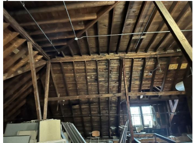
Photo 6: Roof framing of Original Structure as Seen from the Attic
