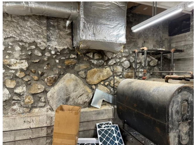
Photo 2: Mortared Stone Foundation Wall in Original Building
