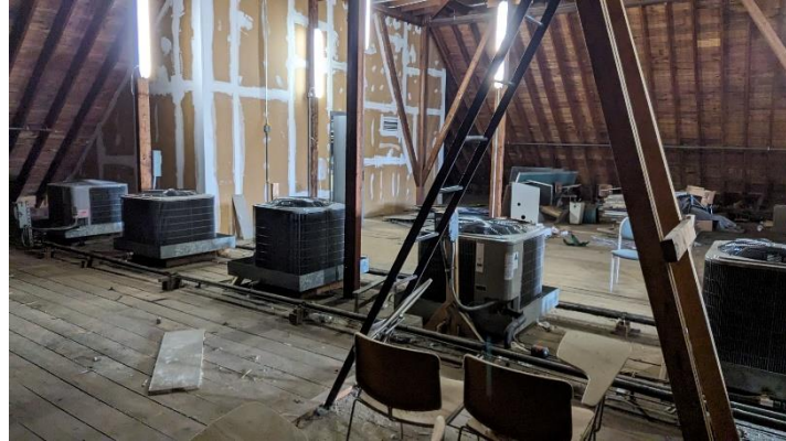
Indoor Condensing Units
