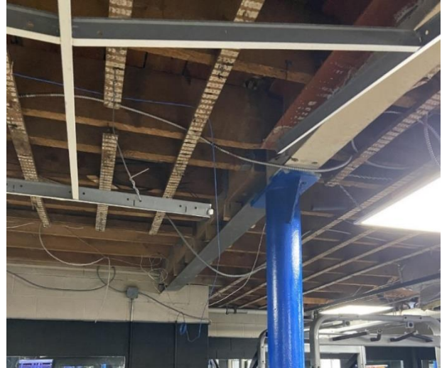
Photo 4: Floor Framing in Original Building as Seen from the Gym
