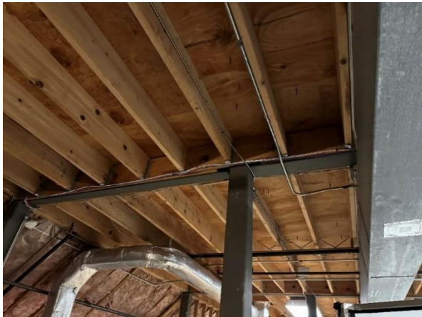
Photo 5: Roof Framing in 1991 Addition as Seen from the Mezzanine
