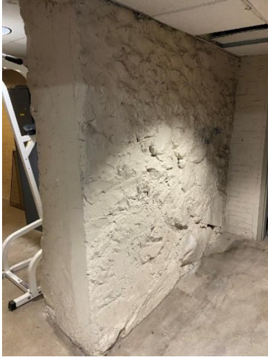
Photo 3: Mortared Stone Foundation Sawcut for Opening to Addition
