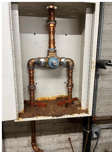
Thermostatic mixing valve
